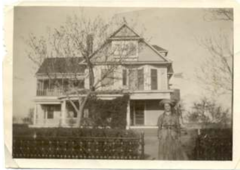
Above: Birdie Cauble E112 is shown in front of the George Clinton Cauble House on Robert E. Lee Road in the 1910s. Image submitted by Richard Cathey Cauble E1162
